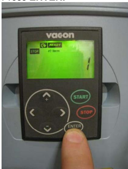
This display screen on the frequency inverter is on a timed window and will return back to the standard “0” if left unattended for too long. Both display screens should be at the same display “page” and ensure both motors are connected before switching to RUN at the control panel.
